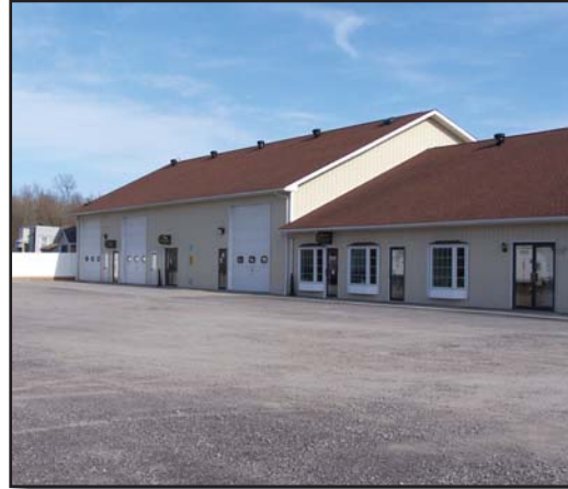
Main Building Side View
